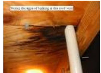
Stains on interior ceilings/walls or mold and mildew growth inside the home may be due to faulty shingle underlayment, allowing moisture to seep into the ceiling and walls.
